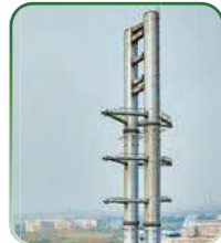
220kV Multi Circuit Tension/ Dead End Dual Pole MSETCL (Maharashtra State Electricity Transmission Company Ltd.), Mumbai
